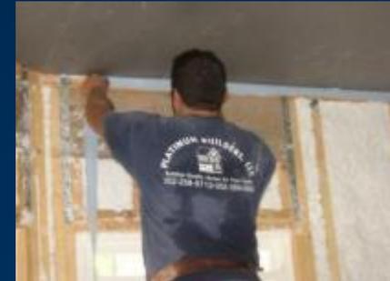
Foam gasket at ceiling/wall joints ensures airtightness
