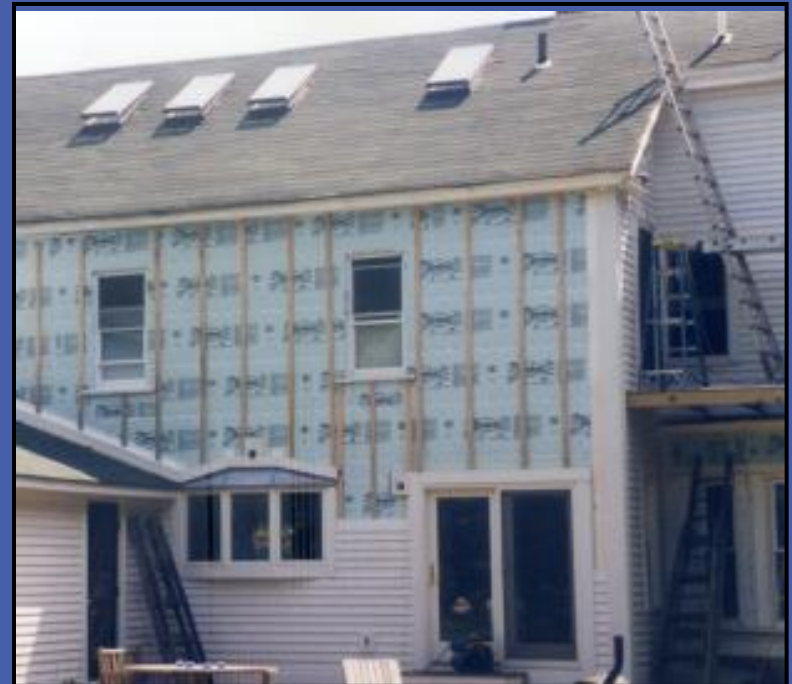
Furring Strips over House Wrap
