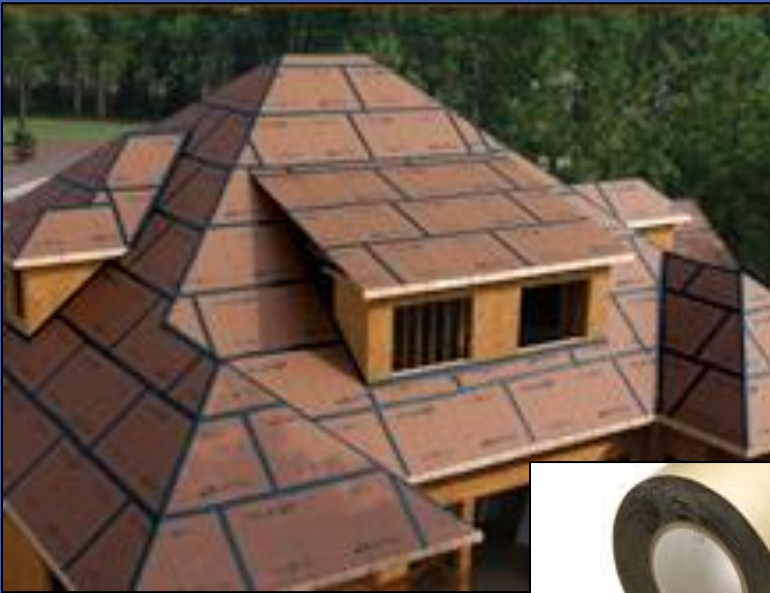
Secondary water barrier on roof
