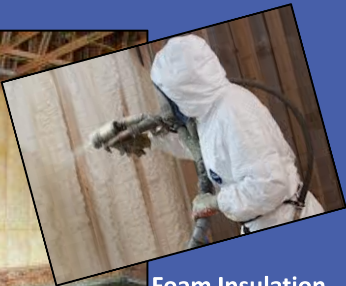
Foam Insulation Frame Wall
