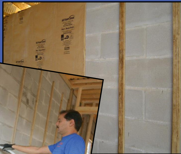
Reflective Insulation Masonry Wall
