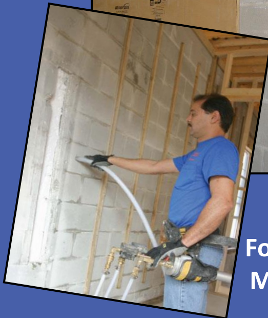
Foam Insulation Frame Wall
