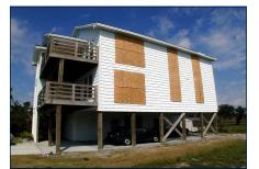
*A quick, effective and easy way* to protect your home is to shutter with plywood board. There are various clips and braces that can be added to hold plywood in place. Insurance companies are not required to provide discounts
